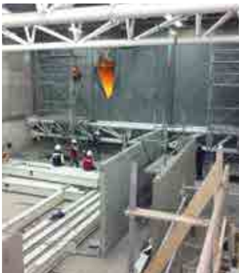
Renovation of Alameda station
