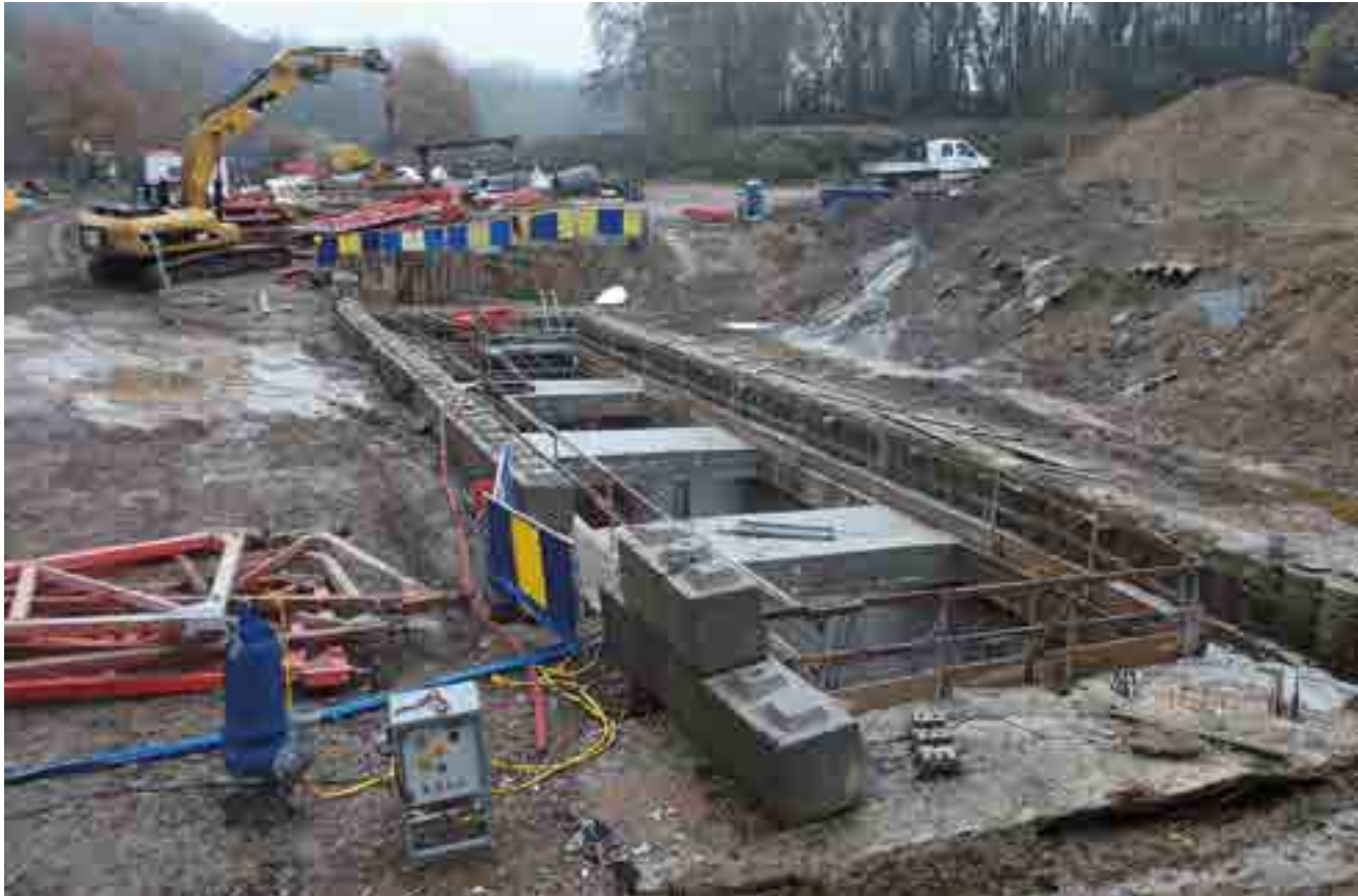
New sewer collector - Verrewinkelbeek Valley (Brussels)
