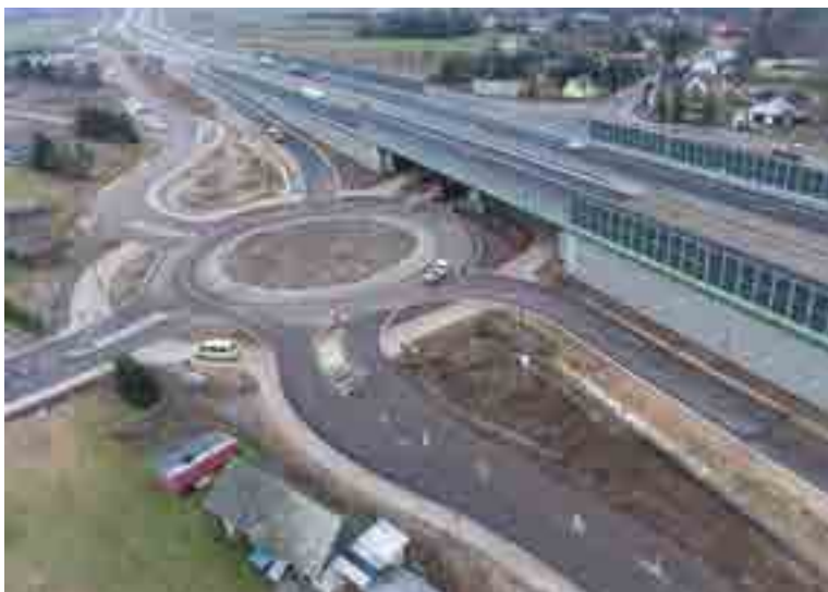
National Road No. 8 linking Warsaw to Białystok, section Wyszkiw - Poreba
