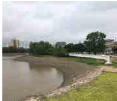
Rehabilitation of the rainwater drainage system of the city of Beira
