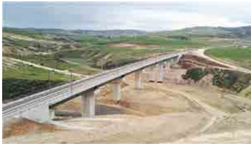
Oued Tlelat - Tlemcen railway line
