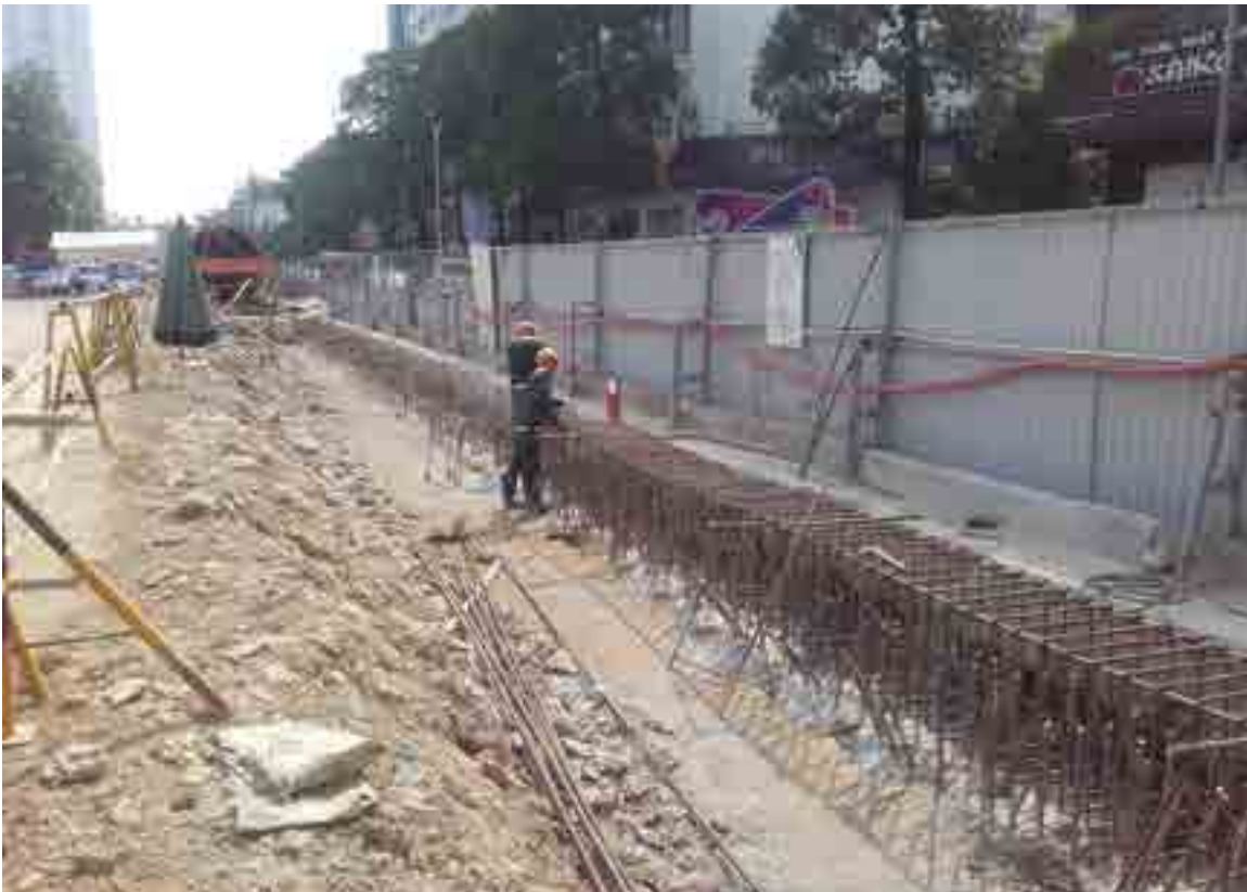
Pilot metro line construction No. 3 - Hanoi
