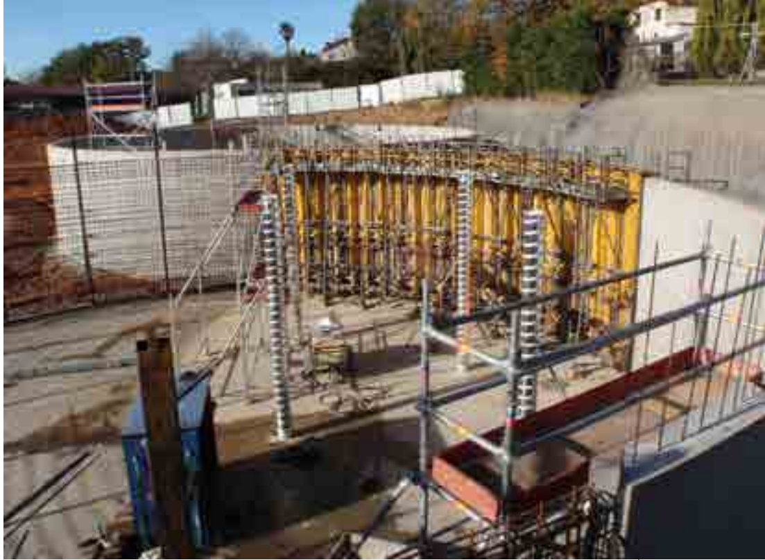
Construction of a drinking water production plant, Albi - France
