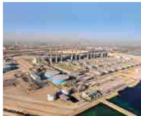
Seawater desalination plant in the Mamelles area of Dakar
