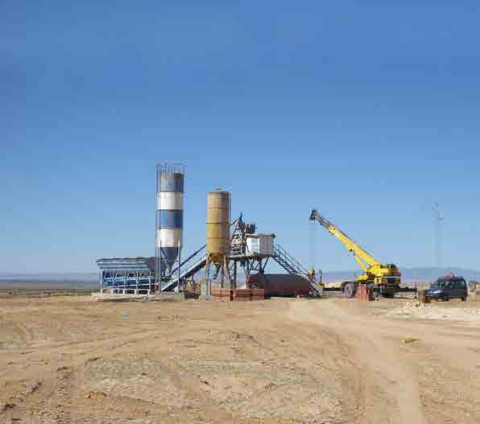
Sewage treatment plant of Sidi Bouzid
