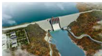
Hydroelectric development project of Caculo Cabaça / Angola
