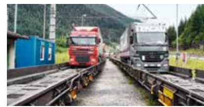
Rail motorway terminal at the Franco-Spanish border (Vitoria-Gasteiz)
