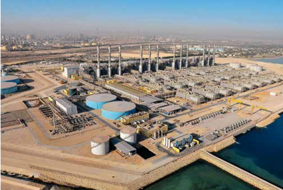
Project of seawater desalination plant in Mamelles – Dakar / Senegal
