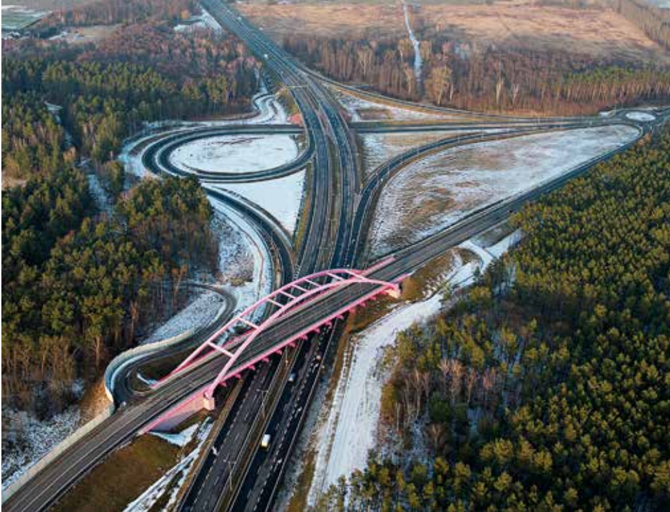
Construction of the second roadway of the Ring Road Międzyrzecz on the expressway S3 km 0+000,00 – km 6+370,00 / Poland
